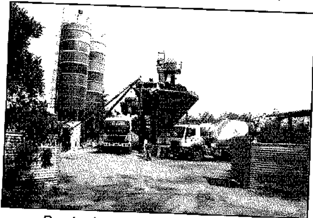
Readymix Concrete Unit at Thanjavur
